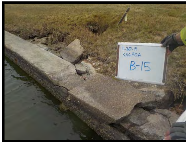
Bulkhead sample point 15.
