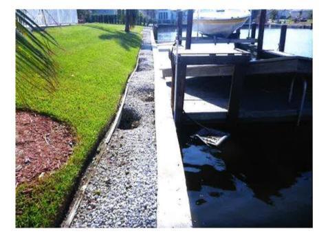
backfill can migrate through openings into the water; frequently occurring after heavy rains.
