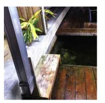
**Panel Joint (Seam) Separation.** Age, uneven exertion of hydrostatic pressure (especially during low tide), or tieback failure can lead to separation between the sheet panel sections.
