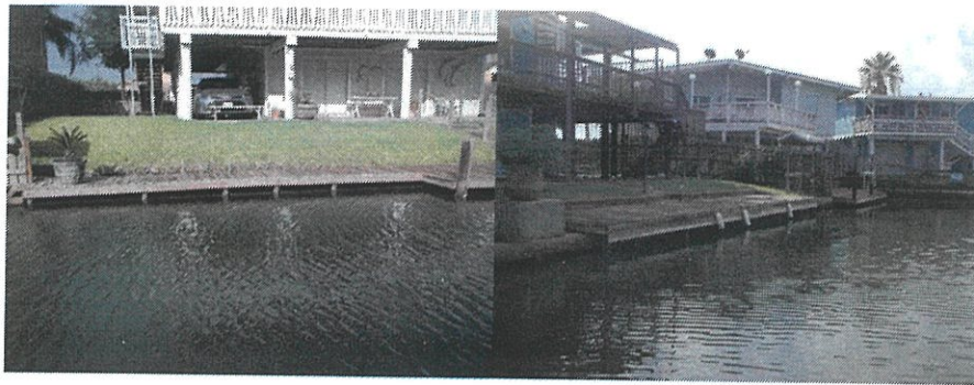
Figure 7: Decking constructed over existing concrete bulkhead
